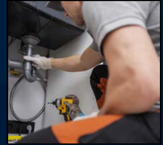
Cert II Plumbing Services 11054NAT
